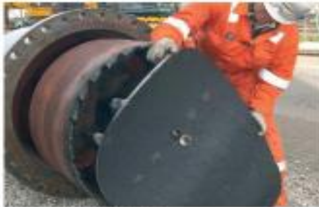
Removal of casing
