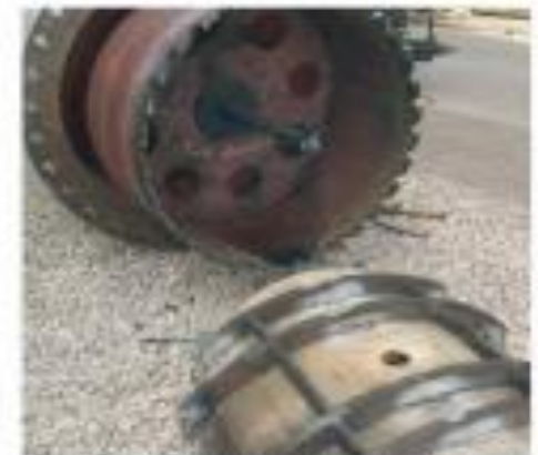
36" casing showing bracing support
